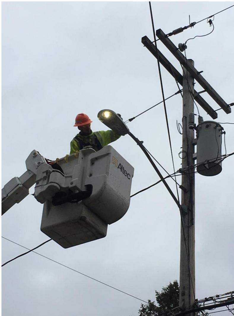
A 100W High Pressure Sodium was converted to a 25W LED on
